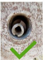
Push a piece of rebar through the dry screw to ensure both screws fit properly together.
